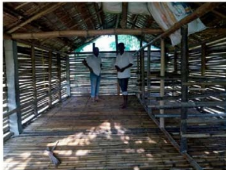
A low-cost Goat Shed made of Bamboo and thatch
